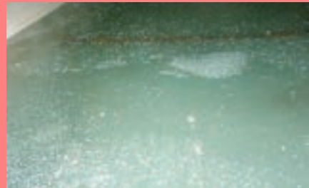
Severe stagnation could indicate that the tank is oversized, or not being used
